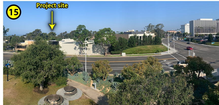
Site Photo 15: East of the Project Site, at Civic Center Park (southwest of San Miguel Drive), looking West.
